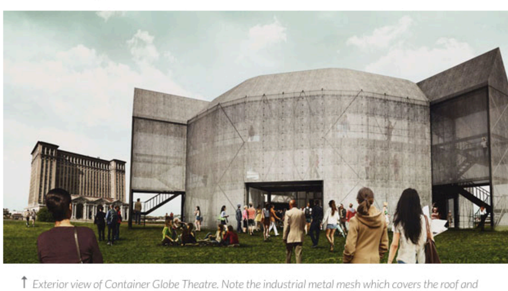
↑ Exterior view of Container Globe Theatre. Note the industrial metal mesh which covers the roof and exterior. The potential for graphics which express the original 1599 structure is enticing.
